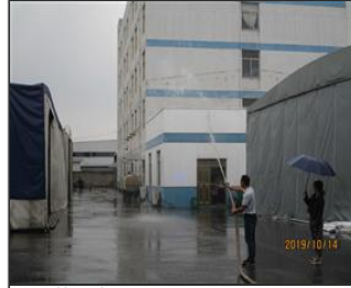
Photo of fire safety equipment Fire water pressure test.JPG
